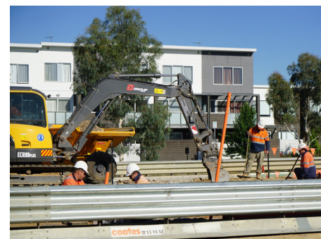
Canberra Metro crews on Flemingington Road
