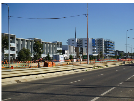
Ground works on Flemingington Road
